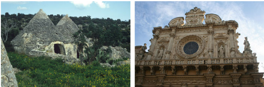
Fig. 2 Examples of the use of carbonate rocks in Apulia: the Cretaceous limestones are used for many churches of “ romanico ” style in the Bari district, and for “ trulli ”, the typical Apulian countryside house (left). Miocene marly calcarenites have been, on the other hand, widely utilized for the “ barocco ”-style churches in Lecce (right), farther south
